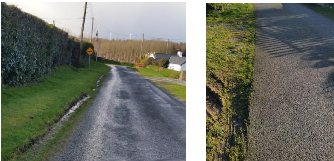
Figure 2-6 Rutting of Road Verge
